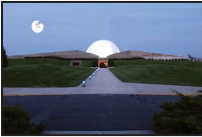
The Armstrong Air & Space Museum, shown here, was designed to accommodate the Astro Theater for multimedia film and sound presentations. The central sphere dominates the entire complex which has earth mounded around the steel-reinforced concrete building. The dome, 560-foot-wide, enhances the futuristic, moon-base design.
